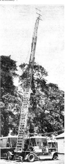
The portable mast in use during the television outside broadcast of the Northolt Derby. It is mounted on a truck and reaches to a height of eighty feet when it is extended.
